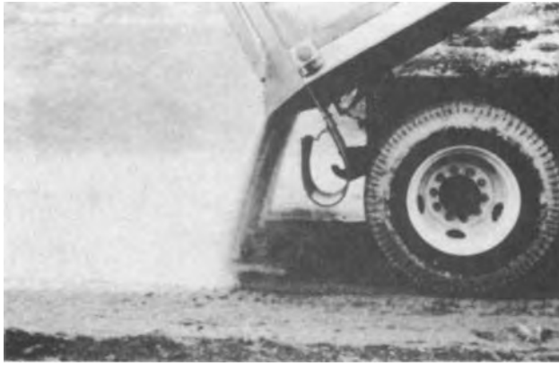
Figure 4-28. Spreading of granular quicklime.
