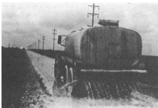
Figure 4-31. Spreading of lime slurry.
