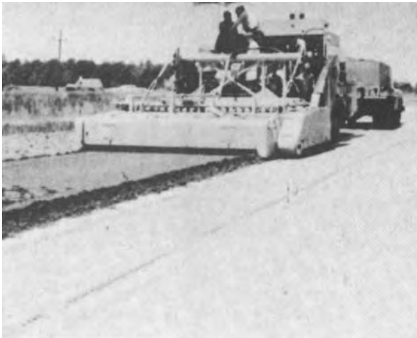
Figure 4-2. Multiple-transverse shaft mixer mixing soil, cement, and water in one pass.
