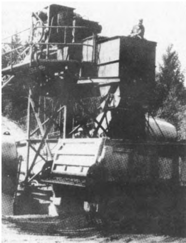
Figure 4-53. Stationary cold-mix plant.
