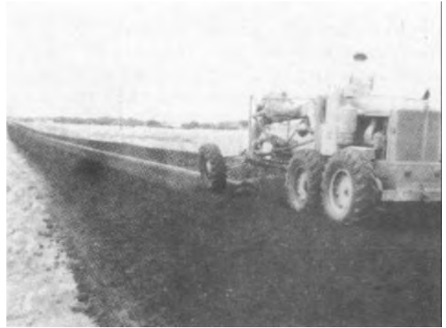
Figure 4-50. Mixing with motor grader.
