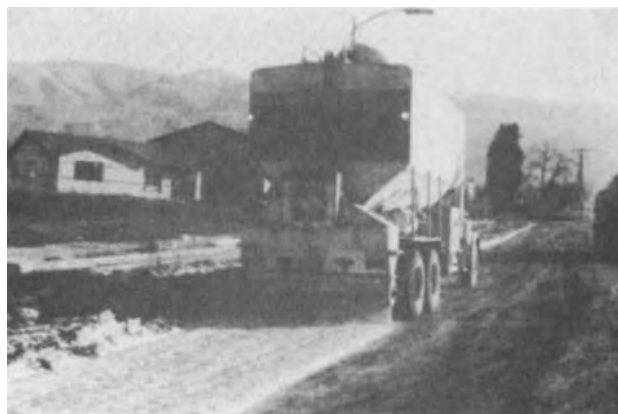
Figure 4-27. Distribution of quicklime from mechanical spreader on city street.
