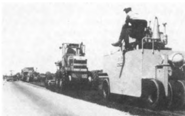
Figure 4-52. Spreading and compacting train.
